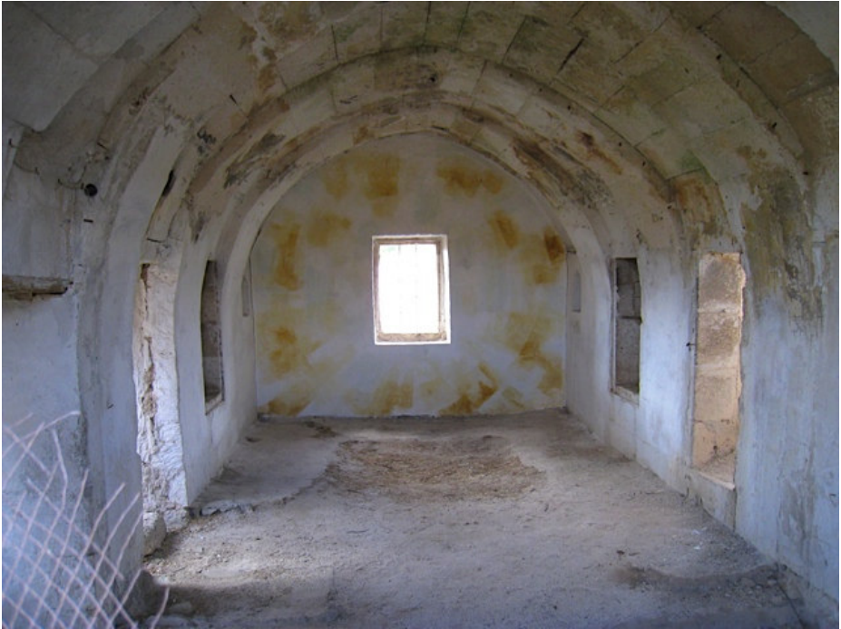
looking in to west wall
