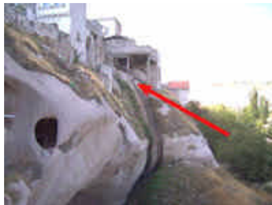
Waste water running in an Ibrahimpasha valley.
